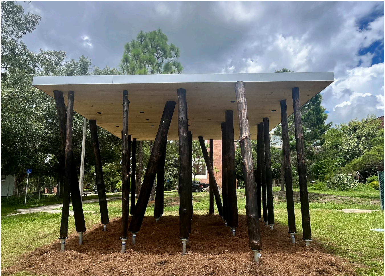
Figure 5. Twenty-eight SYP columns extracted and processed 13 miles from the project site, support a 5-ply SYP-CLT roof of MASS Haptic, a site adjacent to the North Lawn on the main campus at the University of Florida. The pavilion plays host as an outdoor classroom and gathering spot for students and faculty to escape the relentless Florida Sun. Image Credit: Atelier Mey
